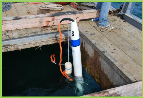
*Photo left: The mooring block was carefully lowered using a length of scrap chain attached to the MVSY winch system. It is essential to lower mooring blocks because they tend to flip over when dropped. The chain will rest on top of the block and probably never be used again.*
